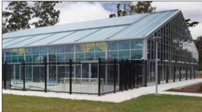
THE AWARD-WINNING SALINAS AQUATIC CENTER IS LEED GOLD CERTIFIED AND FEATURES AN OPENAIRE RETRACTABLE POOL ENCLOSURE. PHOTO CREDIT: LENNY SIEGEL.
