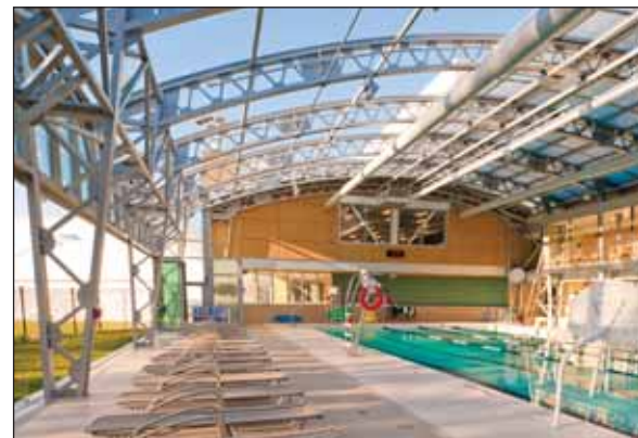
A MODERN RETRACTABLE ROOF ENCLOSURE AT THE TORONTO CRICKET, SKATING & CURLING CLUB. PHOTO CREDIT: ST. GEORGE.
